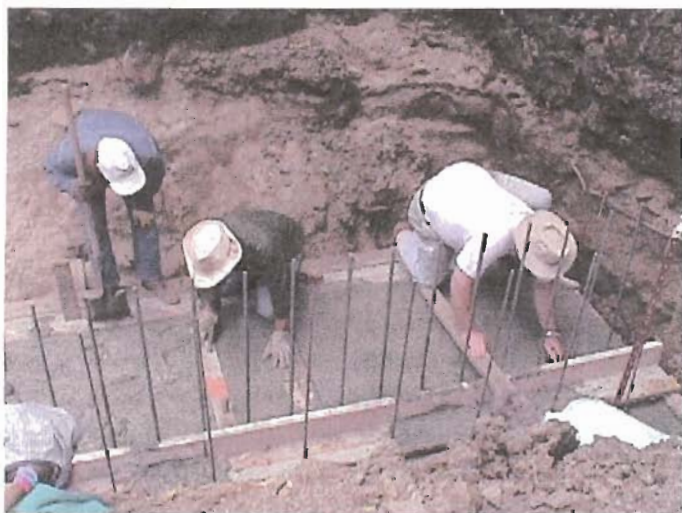
A little foundation work.
