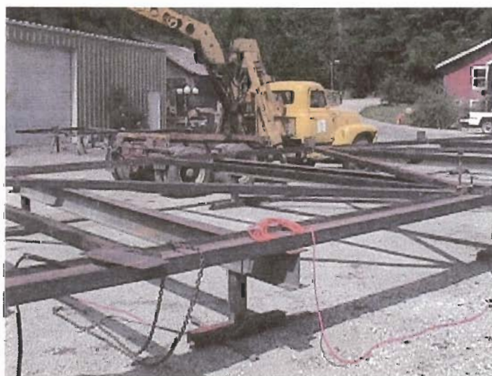
Parts is parts, bridge that is.
