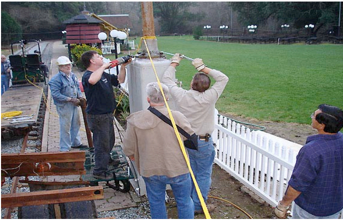
Removing bolts from base of semaphore
