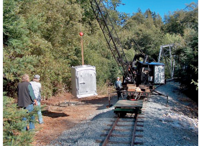
Placing signal base on concrete pad
