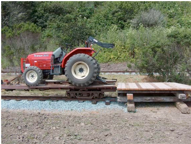
New loading ramp at the train field
