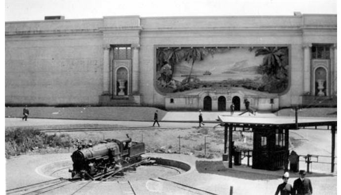
Photo 3 Turntable and ticket booth
