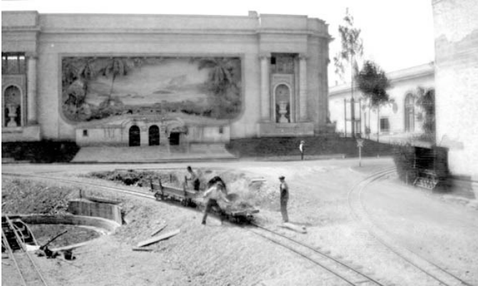
Photo 1 Overfair railway's turntable
