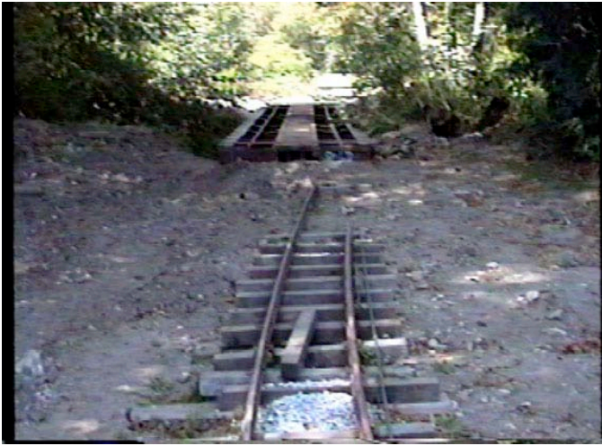
Little Creek Bridge and track approaching, Aug 1992
