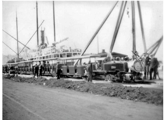
Overfair train passing the boat docking area of the Panama Pacific International Exposition. The train is pulled by the No. 1500 0-6-0T work locomotive. The boat in the background appears to be a passenger boat.
