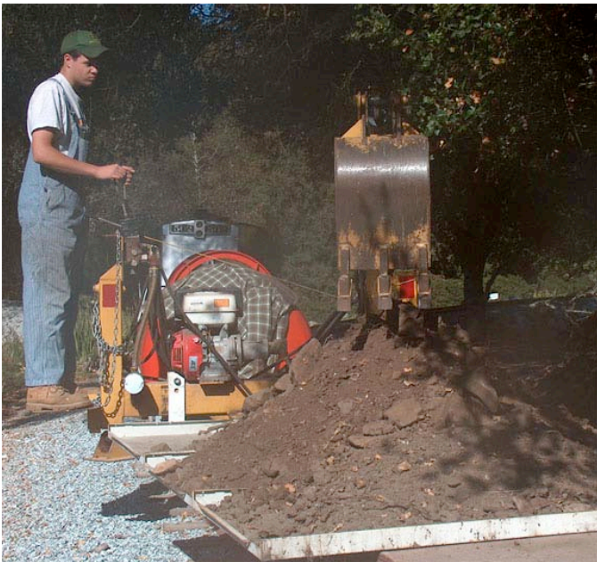
Aaron, ditch cleaning along track
