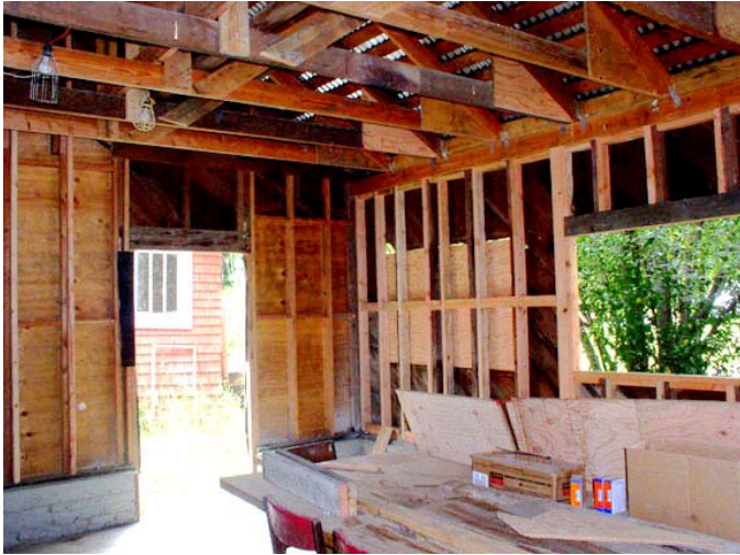
Cal Barn with new wall framing and trusses
