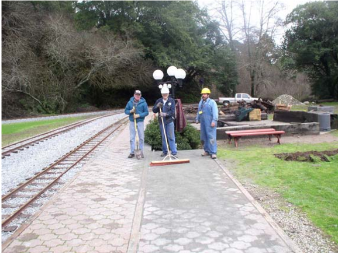
Finishing Station platform
