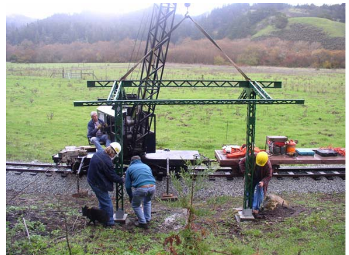
The station at the McNab Grove being set
