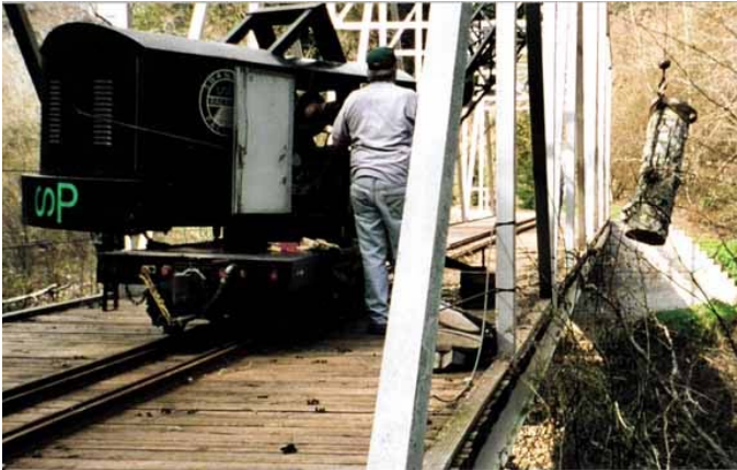
Removing downed tree from creek
