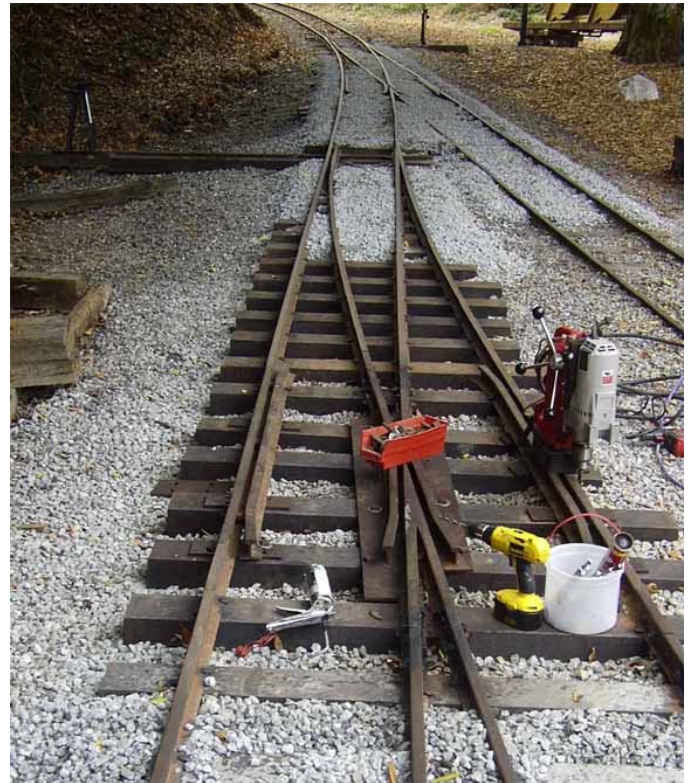
Switch work, replacing ties
