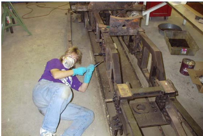
Corrin working on the locomotive 1500
