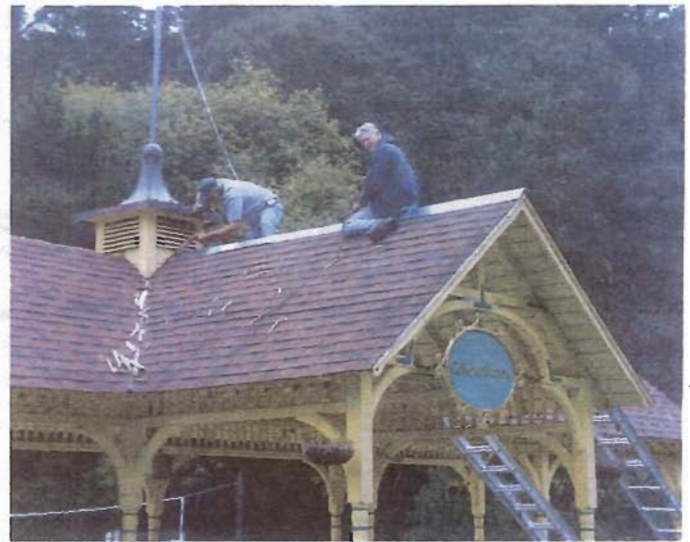
Working on roof
