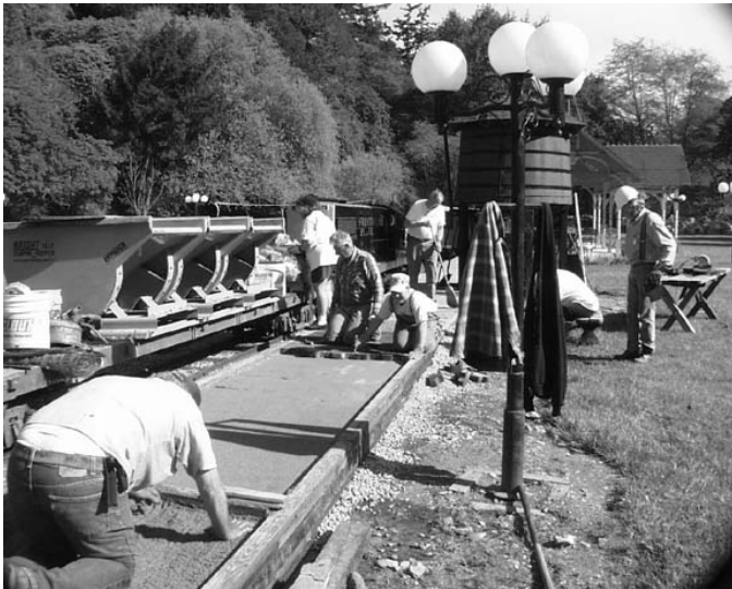
Paver Crew -expanding the loading platform
