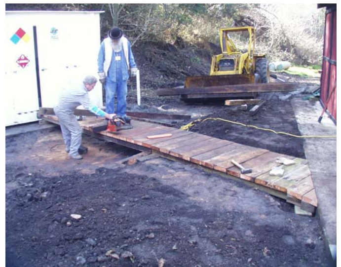
Bridge to oil storage
