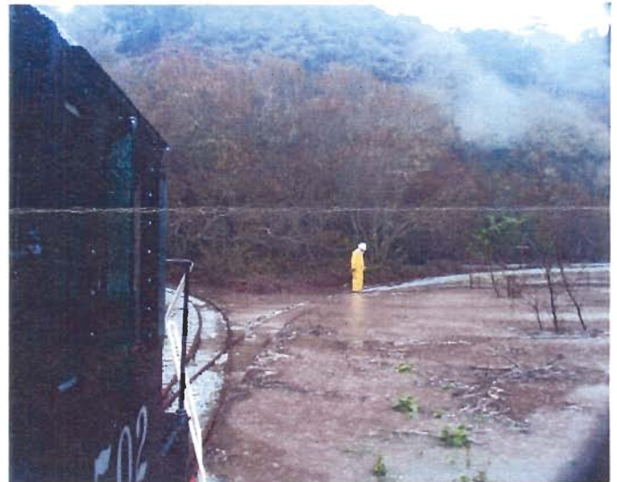
Andy checking track during flooding at the Wye
