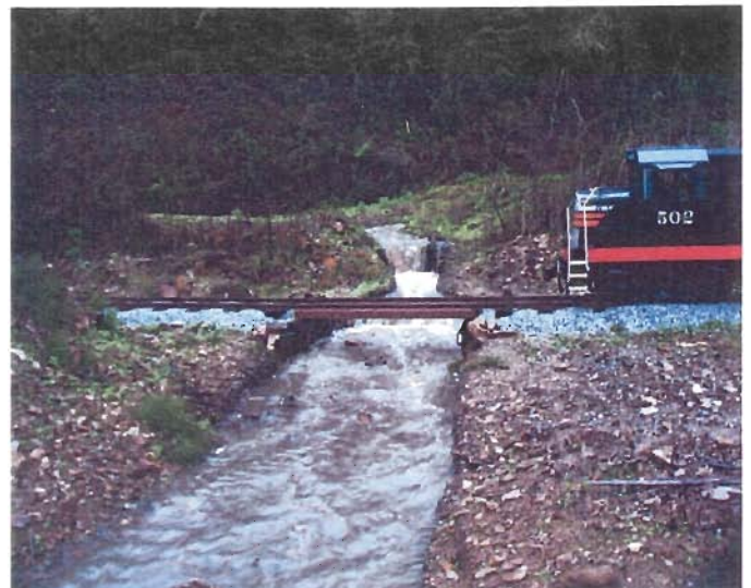
Flow through culvert from McNab Redwood grove
