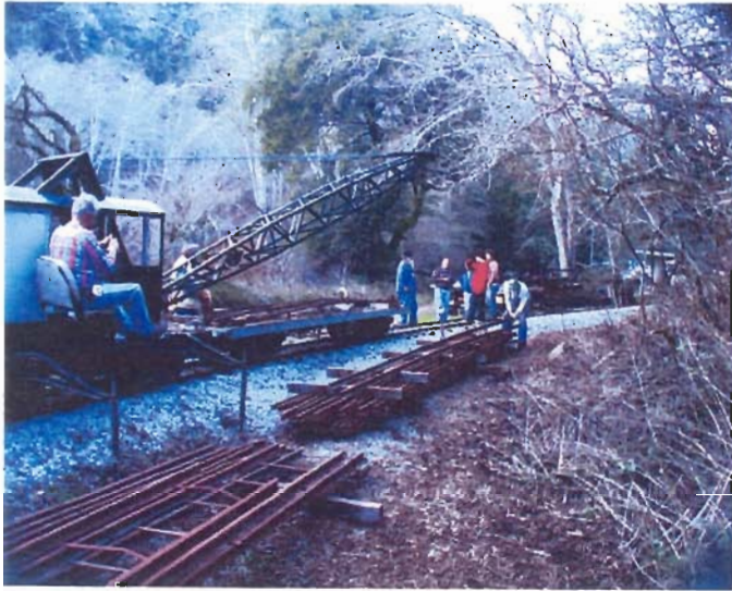
Crew moving rail
