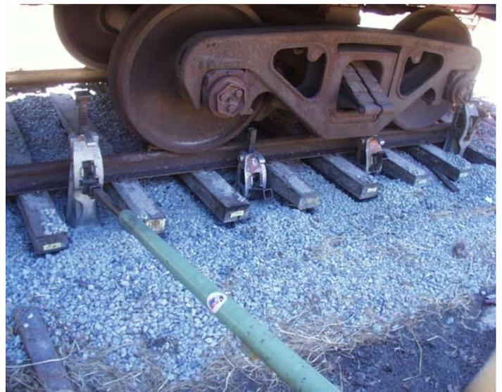
After the new rail was installed we would then lower the caboos back down onto the rail and re-spike the ties. This was a real tedious, not to mention precarious, task in that you are working under the caboose and trucks to remove and replace the spikes.
