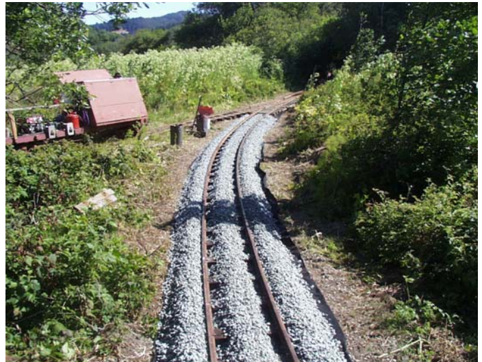
Photo 3 Ballasted Track --- Track once again ready for operation.
