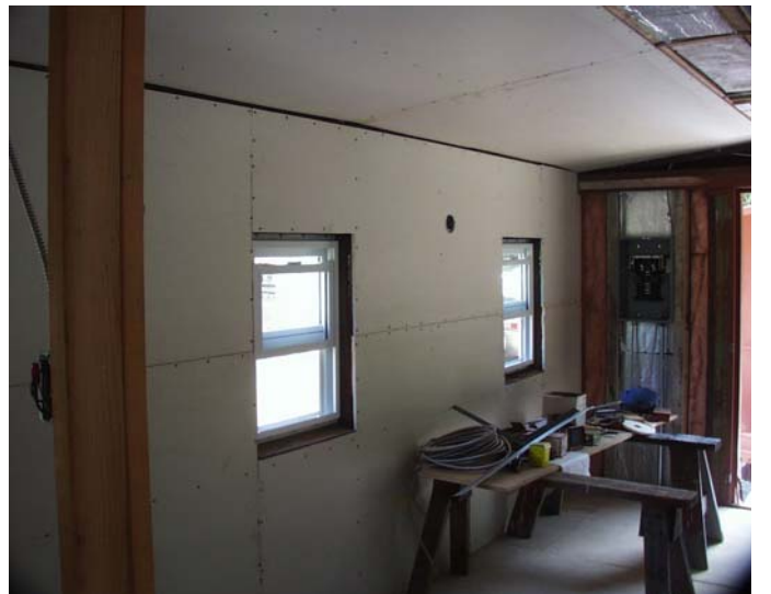
Photo 4 Caboose's Drywall Installed
