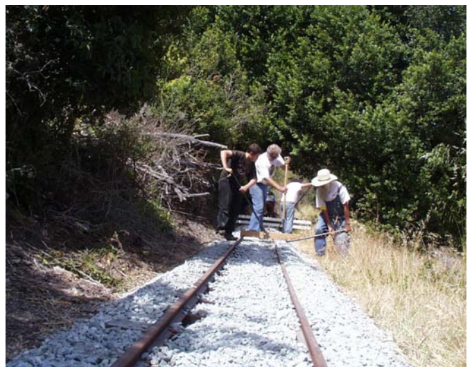
Photo 5 Raising and Tamping Track
