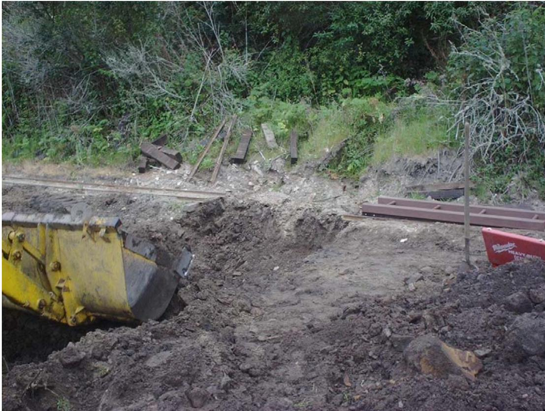
Removing the landslide across tracks and putting in a removable track section so that the next winters rains won't hinder operations.
