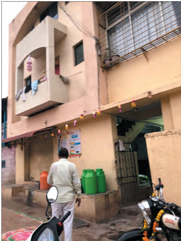
Figure 7: A new three-story courtyard house built of concrete had replaced the traditional one and a dairy is operating from the storefront. The bright green and orange containers are used to collect and ship the milk.
