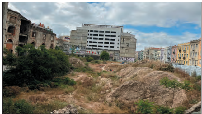
Figure 6: View of the interior of the project block looking south. The historic building shows on the left and the vacant office tower on background. (photo: V. del Rio)
