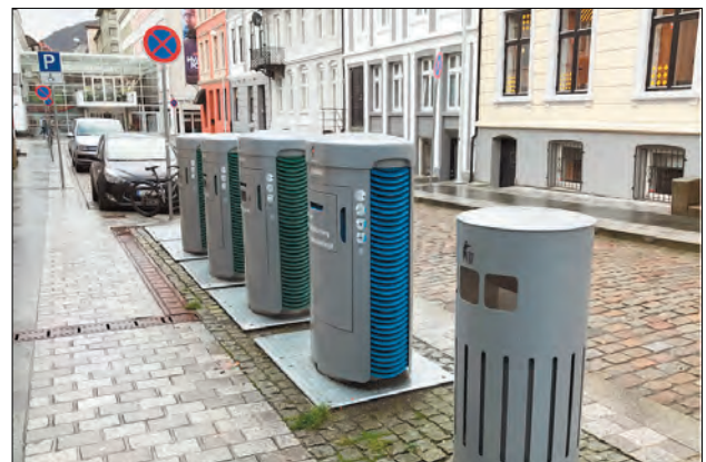
Figure 2: Bergen, Norway has a 7.5 km long vacuum operated smart garbage collection system. (source: https://tomorrow.city/a/from-nocturnal-trucks-to-ai-how-urban-waste-management-is-changing )
