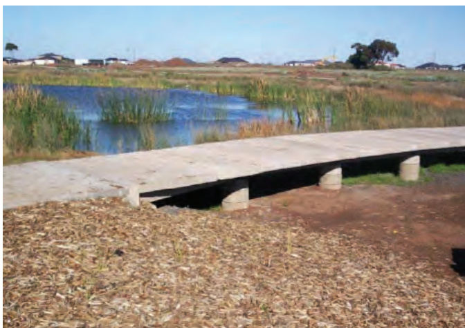
Figure 4.35 Examples of Footbridges
