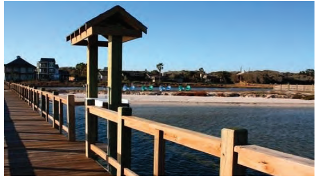
Figure 4.43 Examples of Cleaning Stations on Piers
