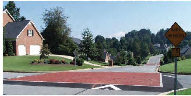
Figure 4.23 Example of Raised and Textured Intersection
