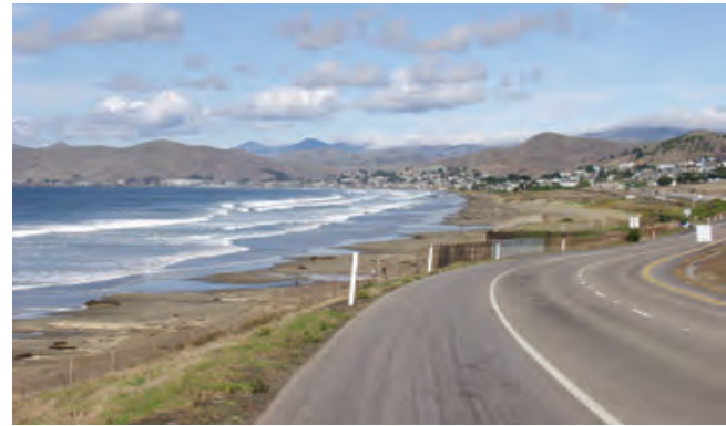
Figure 2.23 Highway 1 south view
