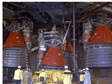
Installation of F-1 engines to the Saturn V S-IC Stage. The nozzle extension is absent from the engine being fitted.
