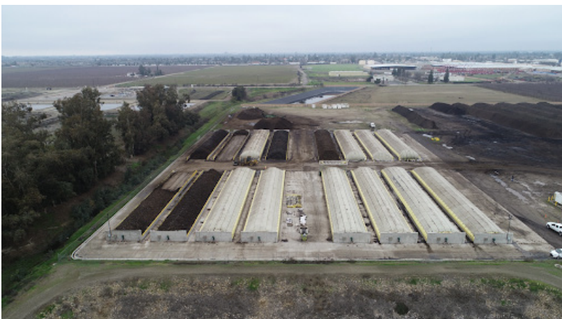
Figures 10 & 11: Kern Composting Facility with GORE covers, processes about 290,000 TPY (145,000 cubic yards)
