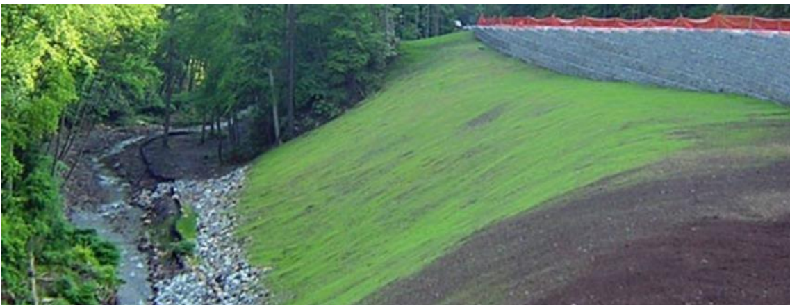
Seeded compost erosion control blanket, photo courtesy of Filtrex
