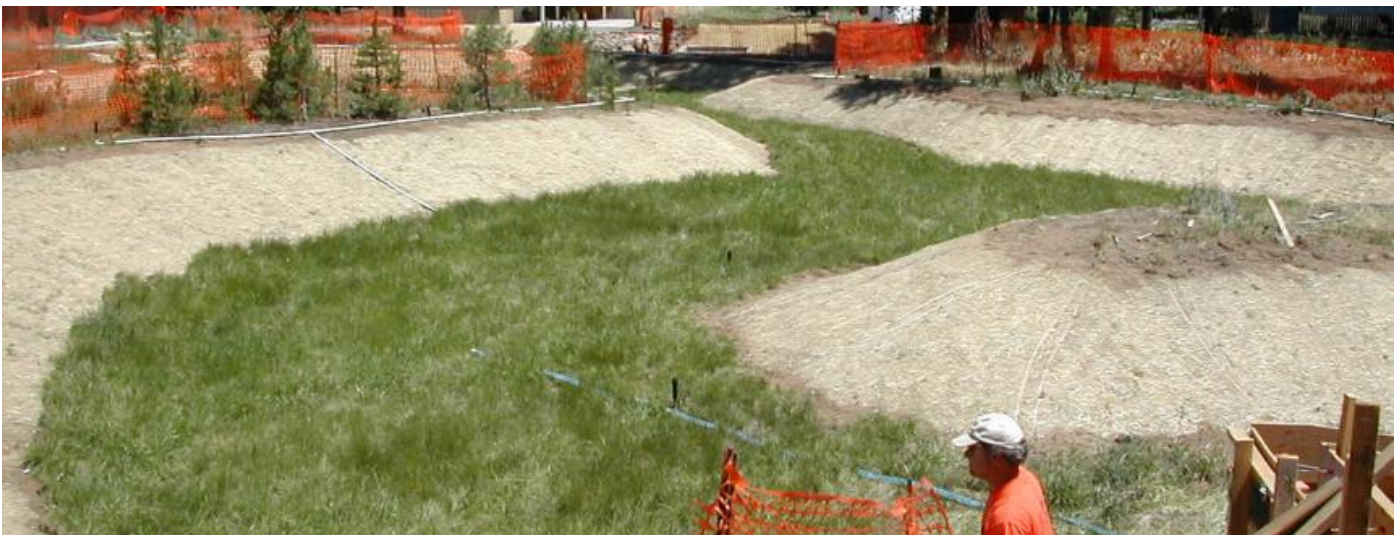
Biofiltration swale, photo courtesy of Caltrans
