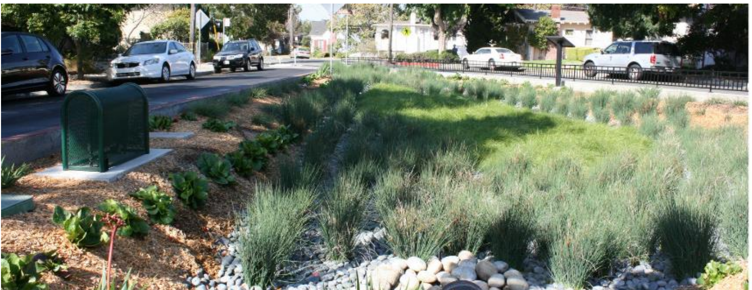
Rain garden retrofit replaced excess asphalt as part of green infrastructure project in Berkeley, photo courtesy of Matt Fabry
