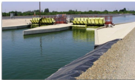
Figure 1. Raceway pond with paddle wheels for wastewater treatment. Lundquist participated in the design of this full-scale facility for secondary treatment only, which was commissioned in 1998 and still operates.
