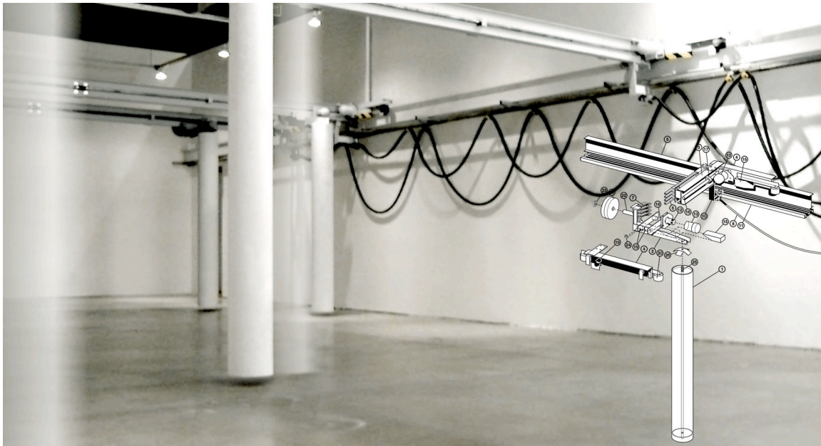
This installation tests a prototype system for reconfigurable architectural space-making elements. In this case, three columns can be repositioned in order to create different spatial relationships with each other and with the walls of the surrounding space. (image: Jones, Partners: Architecture)
