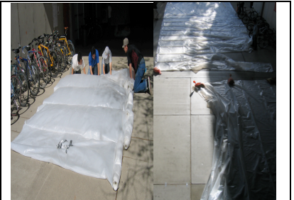
08. Polyethylene Being Rolled up to Hoist Into Place
