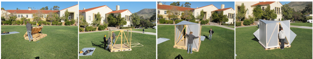
Figure 1: Erection sequence of the flat pack emergency shelter (version 3).
