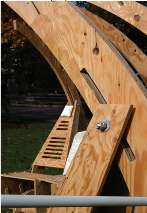
Model as Prototype: model scale based on material thickness. Wood bents measured at scale and then digitally modeled. ▲
