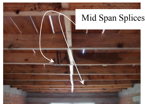
Figure 2: Typical Beam Splice Source: David Lambert
