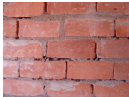
Figure 3: Poor Mortar Joints Source: David Lambert
