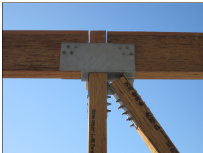
Figure 7: Typical HTBF Connection – As-built Photo
