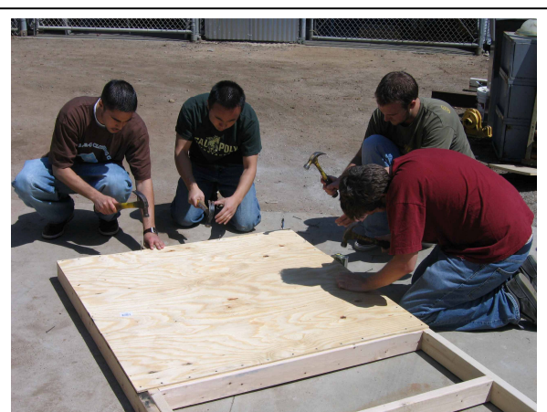
Fig. 6: Applying Sheathing
