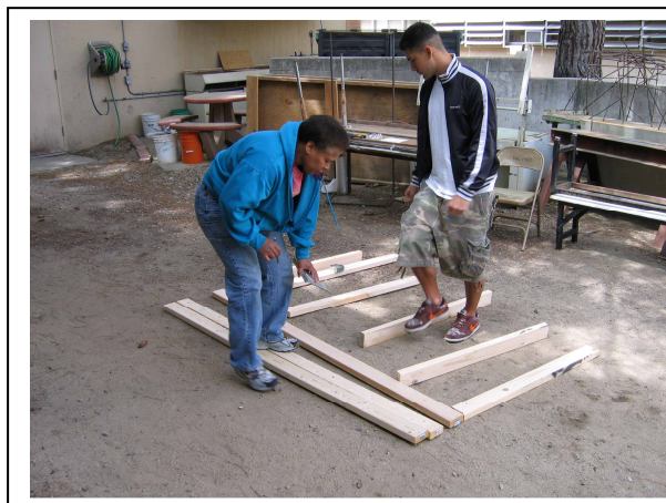
Fig. 2a: Laying Out the Wall
