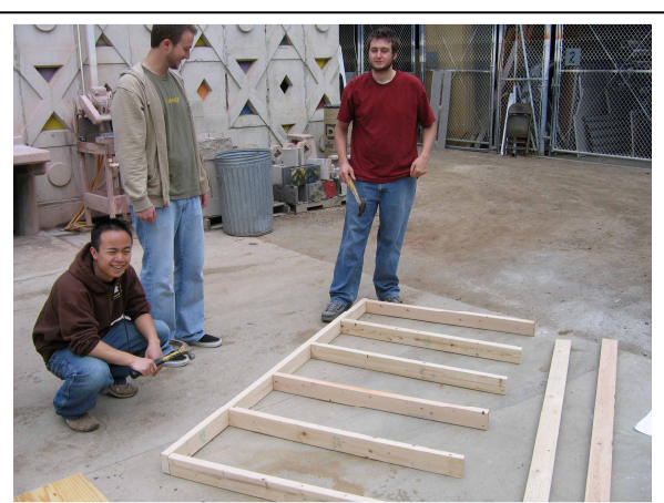
Fig. 2b: Laying Out the Wall
