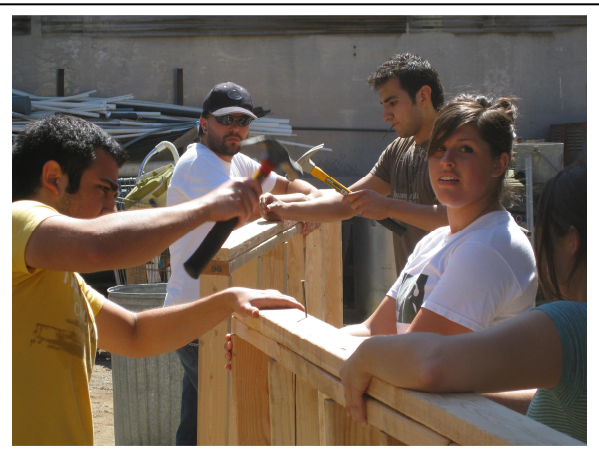
Fig. 5: Double Top Plate Nailing
