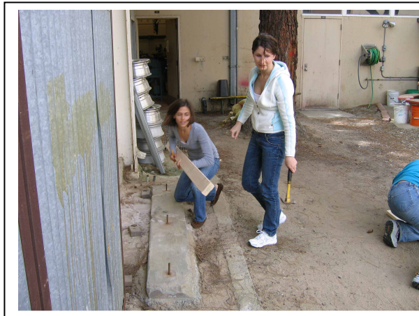
Fig. 3: Measuring for Anchor Bolts
