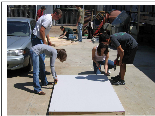
Fig. 6a: Applying Sheathing
