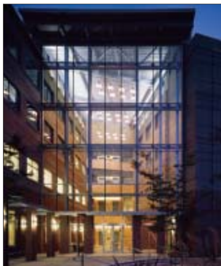
Gladson designed Natural Sciences I (top) and the Calit2 Building (above) at UC Irvine.
